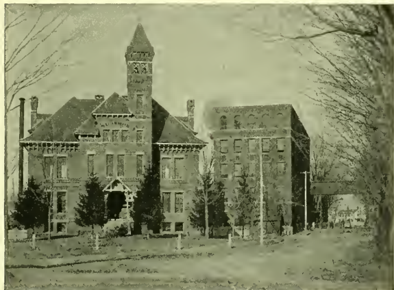
A Chicopee Falls School Building
